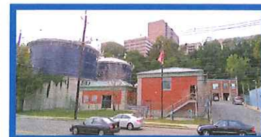
North Bergen MUA Woodcliff Water Treatment Plant
